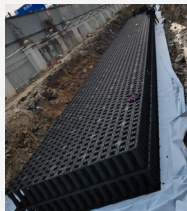
Underground Cistern Construction
